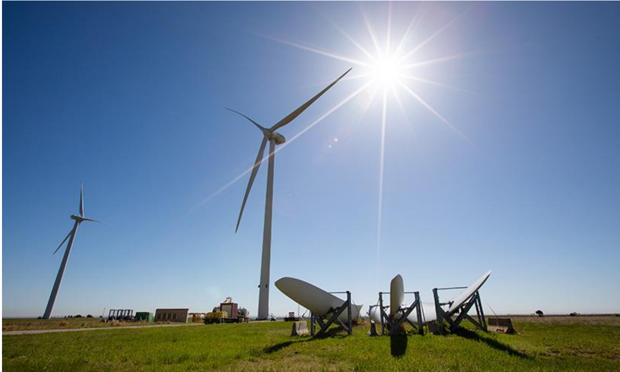
Photo by Werner Slocum, NREL
